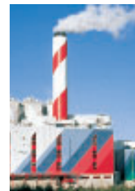
Waste incineration plants.
